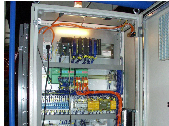
SIMATIC S7-314, In Line modules PHOENIX, Safety relays PILZ
