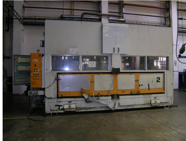
ABB cabin before reconstruction
